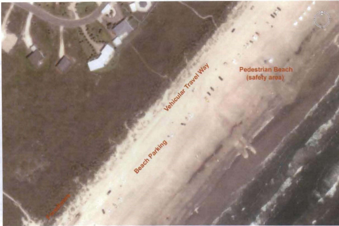
Figure 2. Aerial photograph of a section of public beach in Port Aransas with terminology describing areas (base photograph from http://earth.google.com ).
