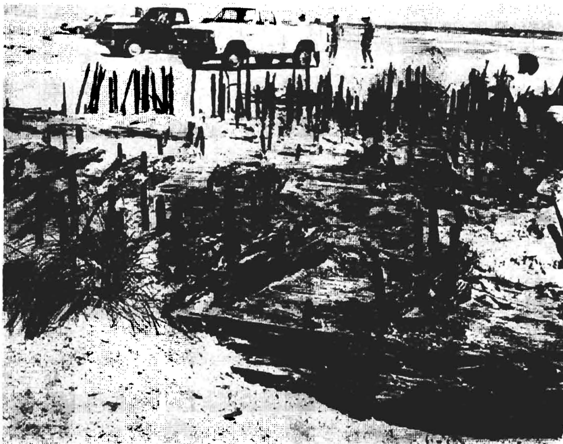
Figure 2. View of anti-torpedo raft centre section, looking northward.
